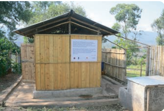
School Sanitation Facility in Shebe District
