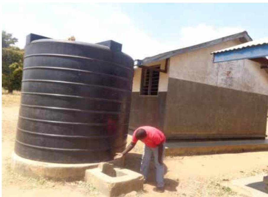
Photograph 1. RWHT with missing tap and gutters
