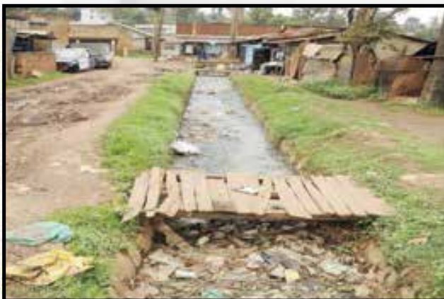
Figure 2: This clogged drainage channel in Kawempe Division will be widened and stone pitched by the project for easy flow surface run off water.
